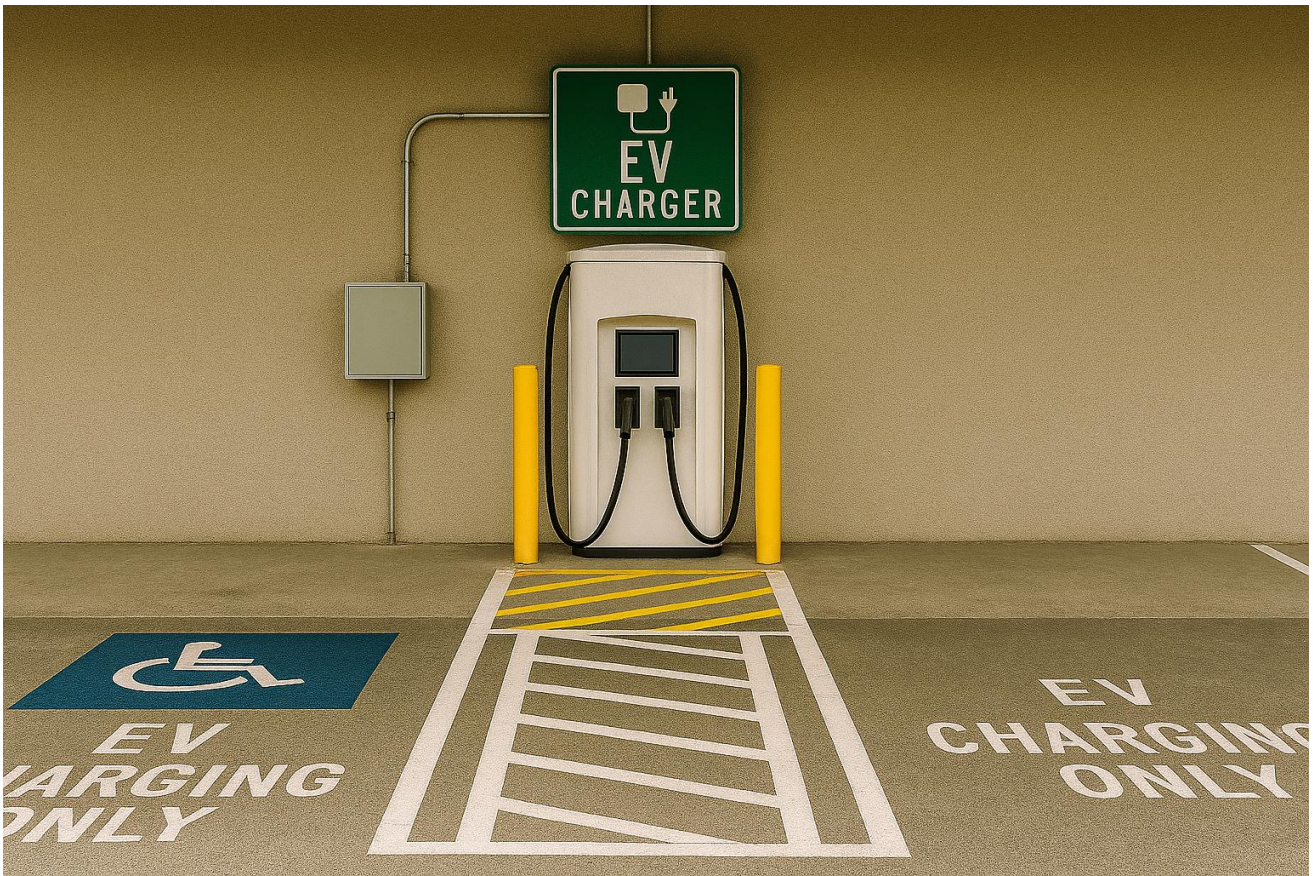
Figure 4-4: Conceptual ADA-compliant EV charging layout showing accessible stall dimensions, access aisle, and compliant reach ranges for charger interface and cable access (AI generated)
