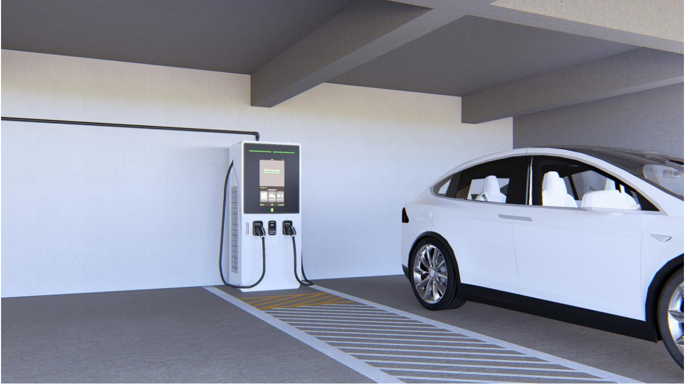
Figure 7-10: Illustration of a dual-port DC fast charger installation showing vehicle positioning, cable reach, and layout within a parking deck environment.
