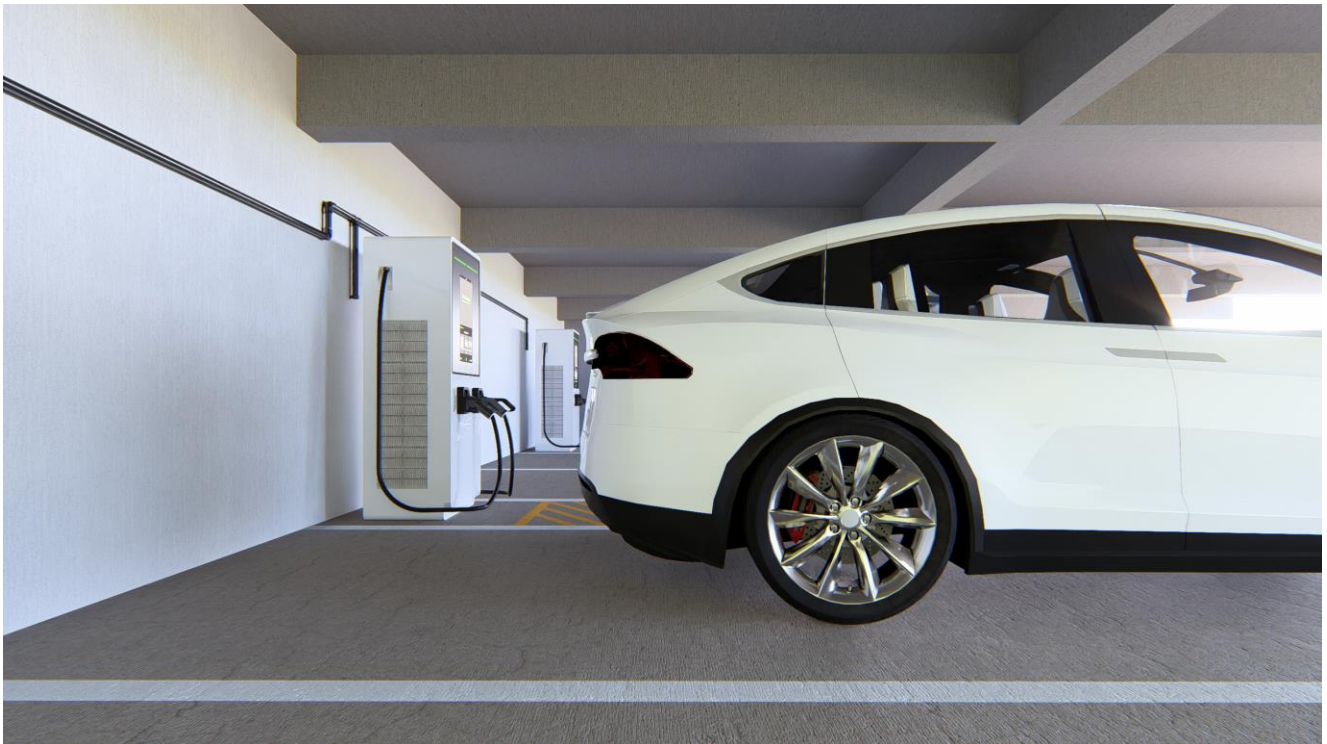
Figure 7-9: Illustration of a dual-port DC fast charger configuration showing charger placement between parking stalls and simultaneous charging of two vehicles.
